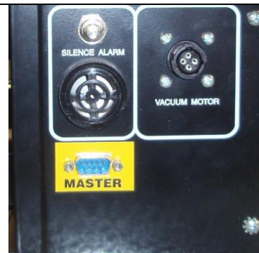
NEW ENDPLATE WITH COMPONENTS INSTALLED
